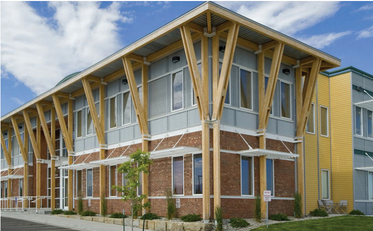
Integrate architectural details with facade articulation. Use a combination of elements such as exposed posts, beams, trusses and brackets.
