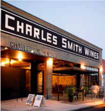
A sign shall be located to fit within the overall context of a building and its site.
